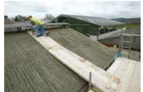
Use boards on fragile roofs
